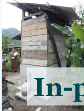
Double-vault urine diversion dehydration toilet, Vietnamese village, Bhutan. Source: WAFLER
